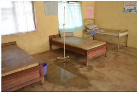
Health facility in Gelegele, Ovia North East LGA, Edo State
