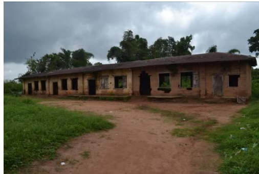
Dilapidated School building in Ikpako, Ovia North East LGA, Edo State
